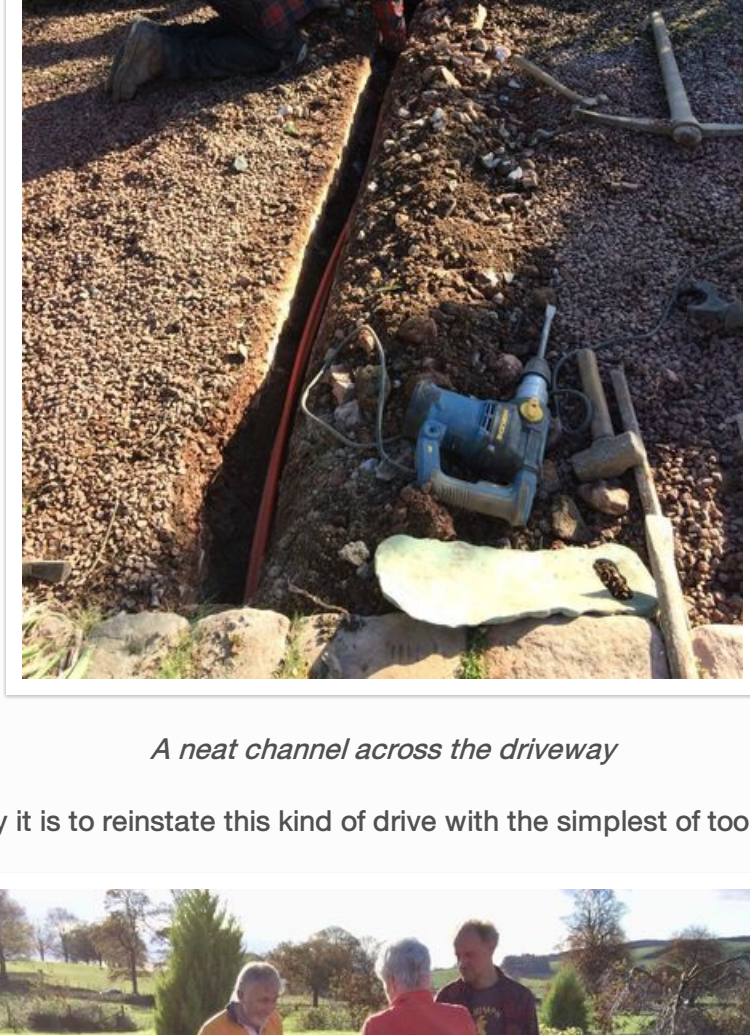
Ducting passes successfully under the wall
